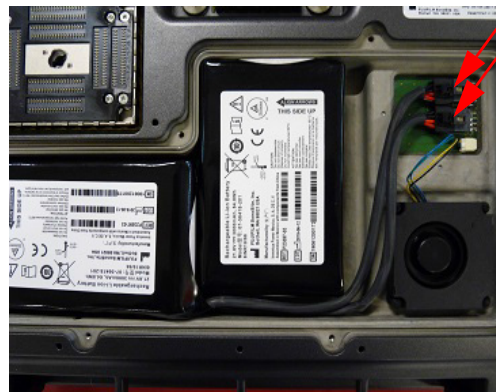
Disconnect Batteries and remove from enclosure
